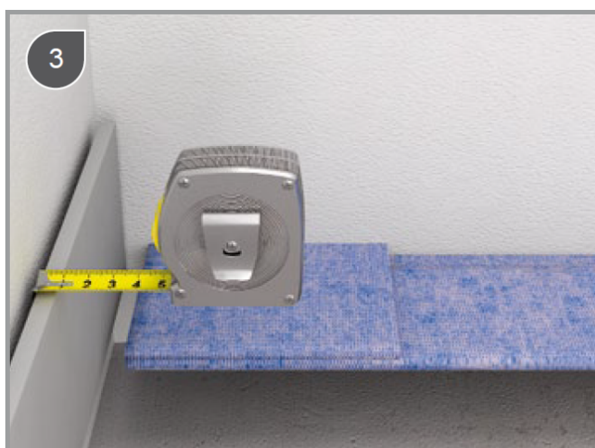
Measure the tile thickness.
