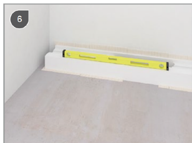
Horizontally position the polystyrene installation block.
