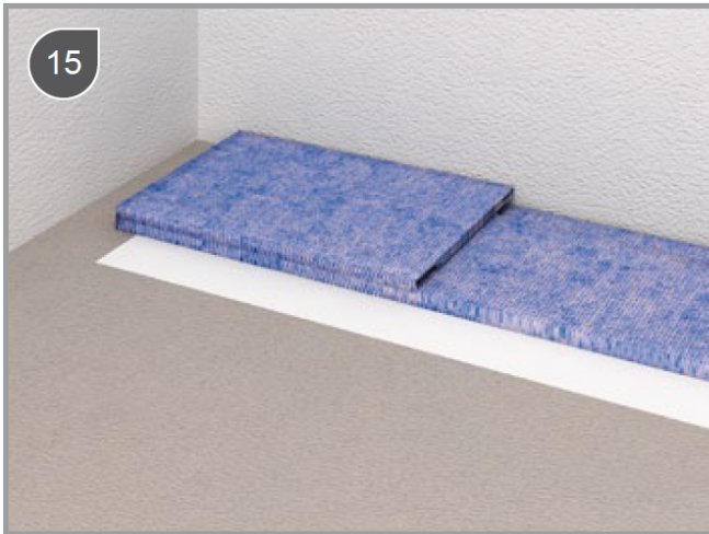
Unpack the waterproof fleece and lap up the wall.
