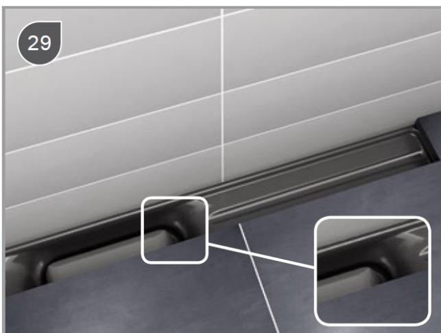
Remove the tile profile.
